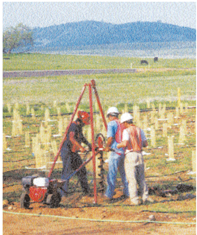
Figure 4. Installing 2 to 3.6 m (6 to 12 ft) cottonwood pole cuttings with a remotely powered Little Beaver™ auger, Yuba City, California.
